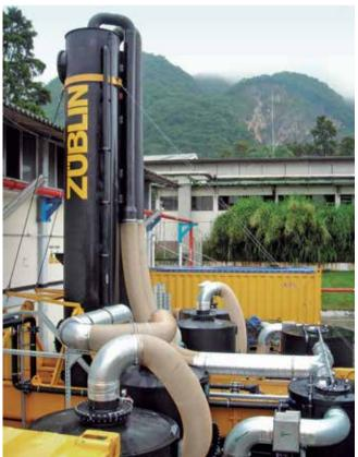
Water Treatment Plant / Desorption system. Stock photo AHK Mexiko
